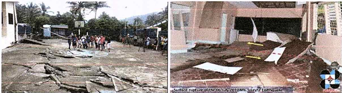
Figure 20. Left: Fault line traversing a basketball court in Ormoc ( www.interaksyon.com , 2017). Right: A school building above a fault line in Leyte)
