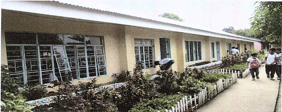
Building 2 showing the casement type window at the left end of the building
