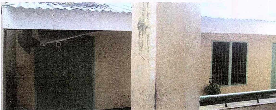
Building 8. Showing the damage portion due to the construction of the adjacent building.(Building No.
