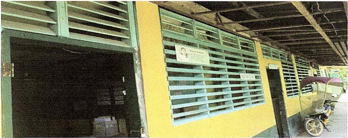
Building 11. Shown in the picture is the wooden grills on windows and the deteriorating condition of the ceiling.
