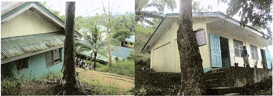
Figure 29. School buildings along slopes (L) School building along slopes in Sta. Rita National High School (Low susceptibility to rain-induced landslide); (R) Sua National High School (High susceptibility to rain-induced landslide).
