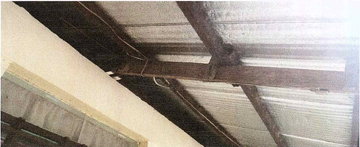
Shown in the picture is the wooden truss and wooden purlins as well as the ceiling of Building 5.
