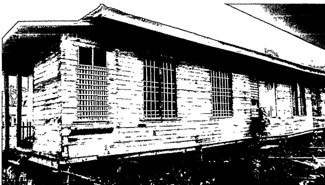
Figure 40: Typical fire risky wooden structures (San Fernando NHS Administration Building).
