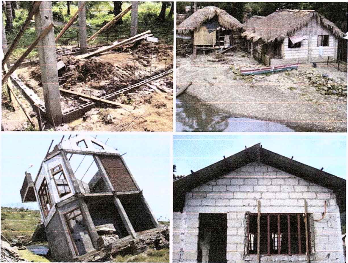
Figure 9. Some common building design issues in the Philippines (Top-Left: poor foundation/swampy; Top-Right: bad location; Bottom-Left: rigid structure in liquefaction zone; Bottom-Right: poor structural condition) Source: GTZ, 2008
