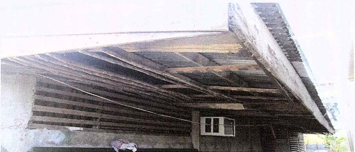
Picture shows the damage ceiling of Building 10.
