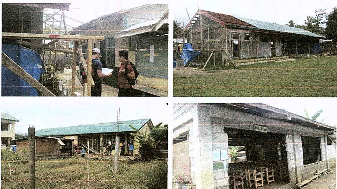
Figure 52. Buildings without construction safety measures. Top Pictures: Under construction buildings of Calapi NHS with no construction safety measures. Bottom Left: On-going construction at QQSAS NHS without construction safety measure. Bottom Right: Utilized unfinished building of QQSAS NHS.
