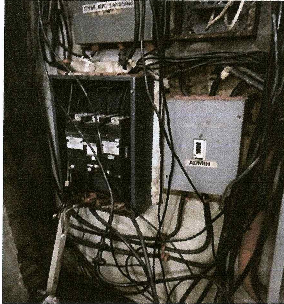
Feeder circuit breaker
